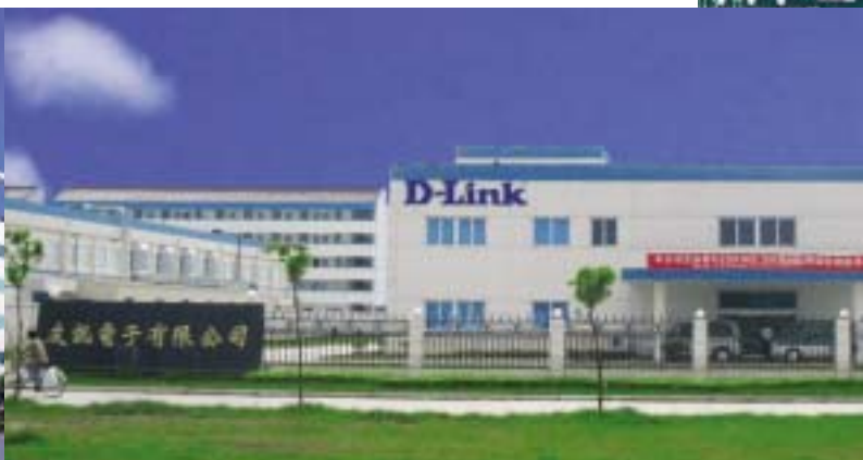
The Wujiang manufacturing facility has a total floor space of 70,500 square feet
